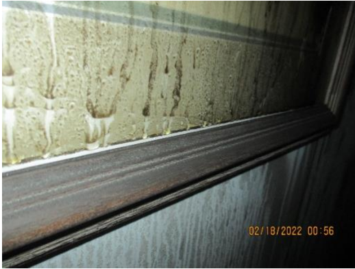
Fig. 10 Condensation streaks of glass
