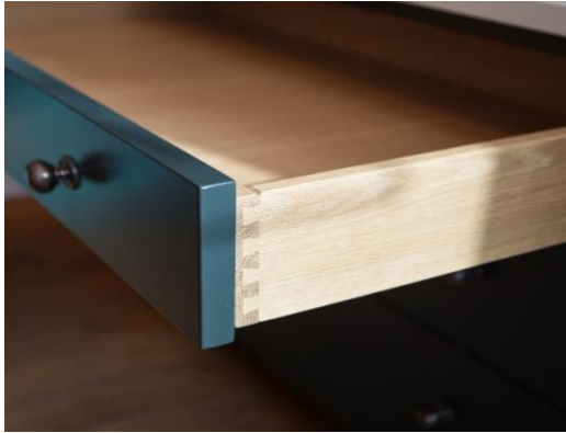
Fig. 4 Dovetail joinery
